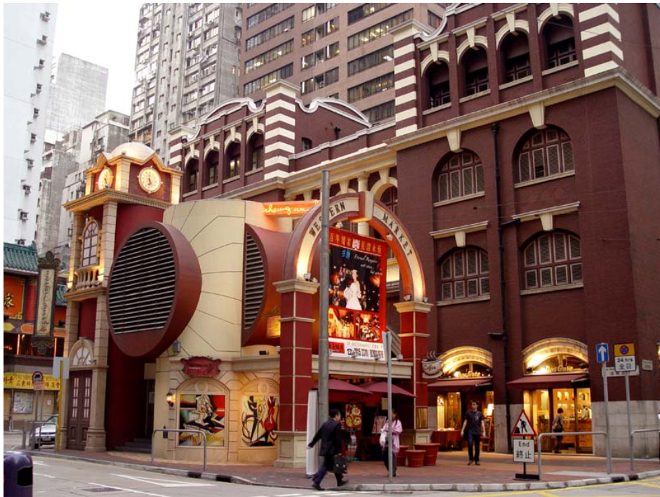
Figure 1: Ventilation facilities of MTR Sheung Wan Station of the Island Line are articulated to blend with the adjacent building.
