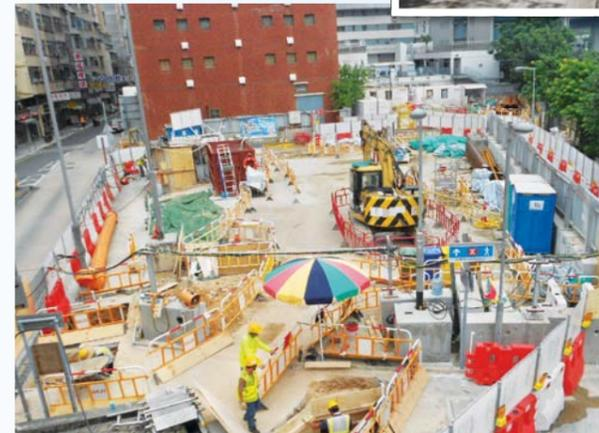
Public utilities located underneath Winslow Street Playground and Car Park are diverted to make way for the construction of approach tunnels to the north of Hung Hom Station.
