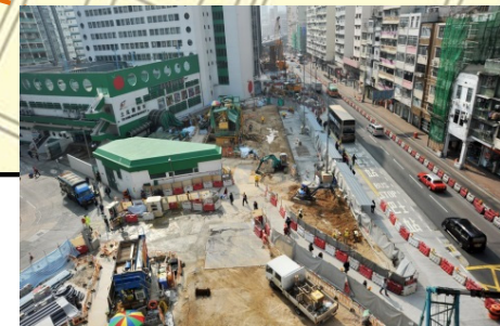
Existing works area at Ma Tau Wai Road.
