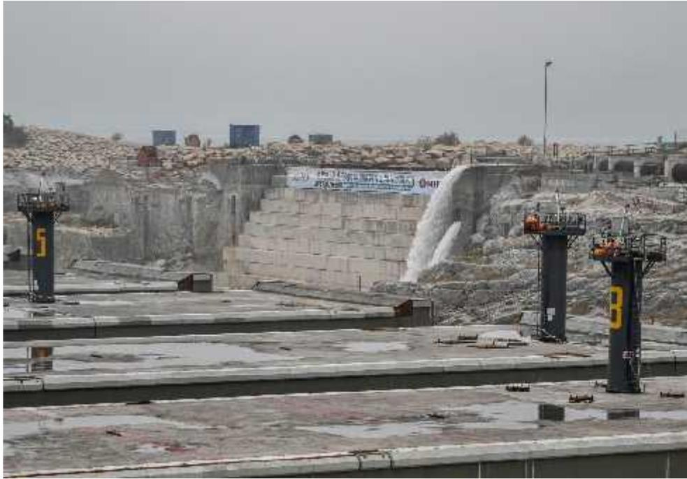
3. Each of the Immersed Tube Tunnel pre-fabricated units will be lowered to the seabed of Victoria Harbour one by one, to form Hong Kong's fourth railway harbour crossing.
